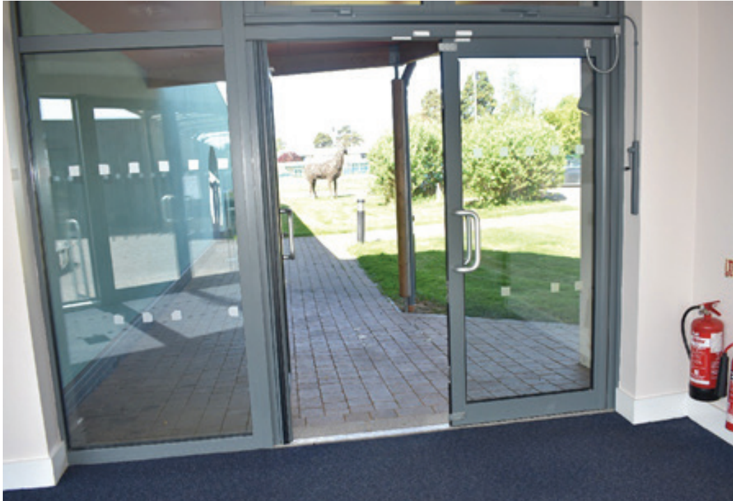
Primary exit door
